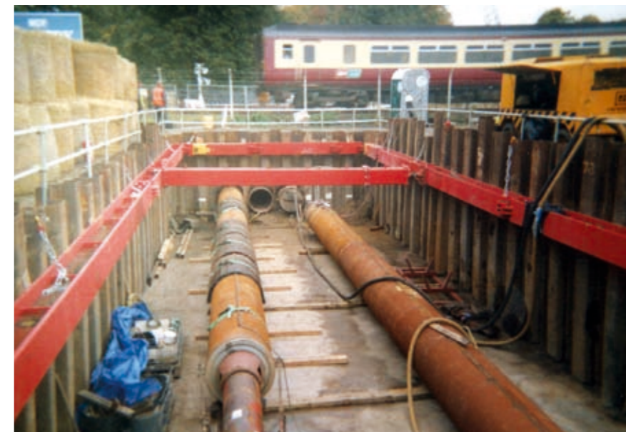
Further preparation showing additional soundproofing and uninterrupted Carlisle bound train.
