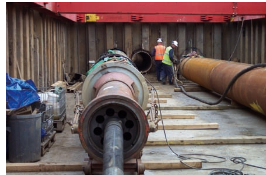
Pipe number 3 ready for ramming and awaiting nighttime possession.
